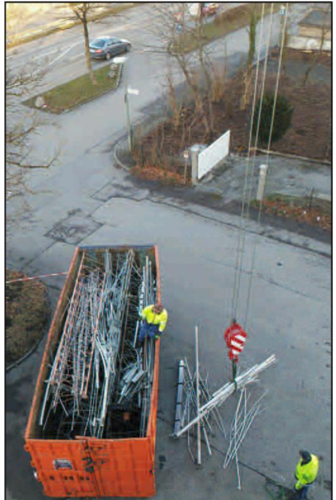
Photos C-F: An unusually severe mid-December storm destroyed the DL1A contest station towers and antennas that were located about a 30-minute drive west of Munich, Germany. Pictures show the towers and antennas before and after the storm. According to an account posted on the DL1A website, a guy wire on the main rotating tower snapped and the falling tower took out the other towers. Fortunately, no injuries resulted. DL1A was hosted by DJ6ZM and the towers were built on the roof of a furniture company. The station is QRT "until a new location is found." (Photos courtesy of DL1A.)
