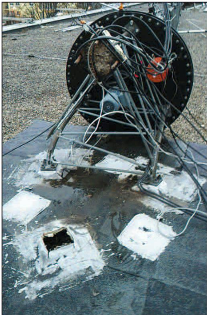
Photos C-F: An unusually severe mid-December storm destroyed the DL1A contest station towers and antennas that were located about a 30-minute drive west of Munich, Germany. Pictures show the towers and antennas before and after the storm. According to an account posted on the DL1A website, a guy wire on the main rotating tower snapped and the falling tower took out the other towers. Fortunately, no injuries resulted. DL1A was hosted by DJ6ZM and the towers were built on the roof of a furniture company. The station is QRT "until a new location is found." (Photos courtesy of DL1A.)
